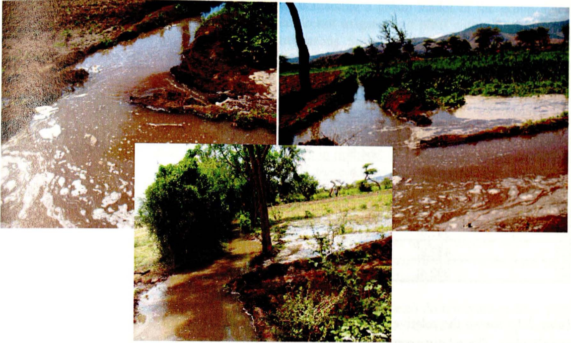
Figure 3.3a b, c over topping of the main canal
